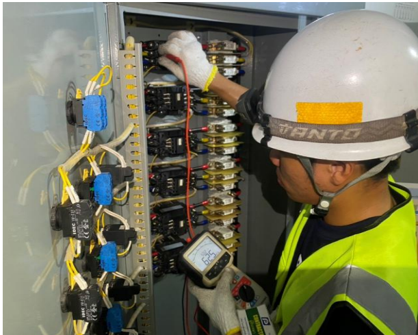
INSULATION TEST
