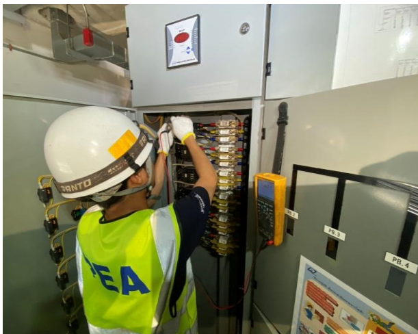
CAPACITOR TEST
