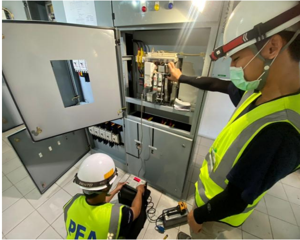
ACB TRIP UNIT TEST
